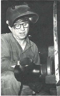
George Grizio prepares for a welding job on a weld neck flange in the pipe shop.
