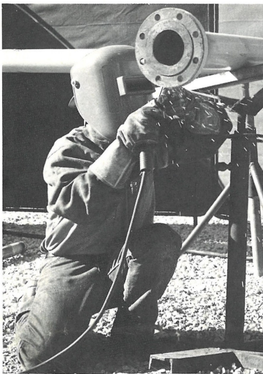
The man behind the mask is Leroy Ducommun. Leroy is welding a flange to a pipe section.
