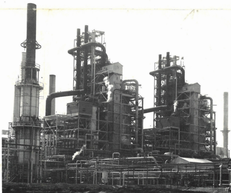
LET'S GET CRACKING. Cat Cracker No. 1 (right) is back up and running after scheduled maintenance. Prior to the shutdown, CCU-1 set a Shell record for continuous operation.
