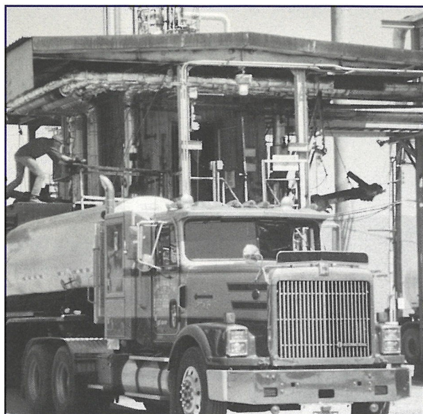
Planned improvements will reduce waiting time at the Asphalt truck loading rack.
