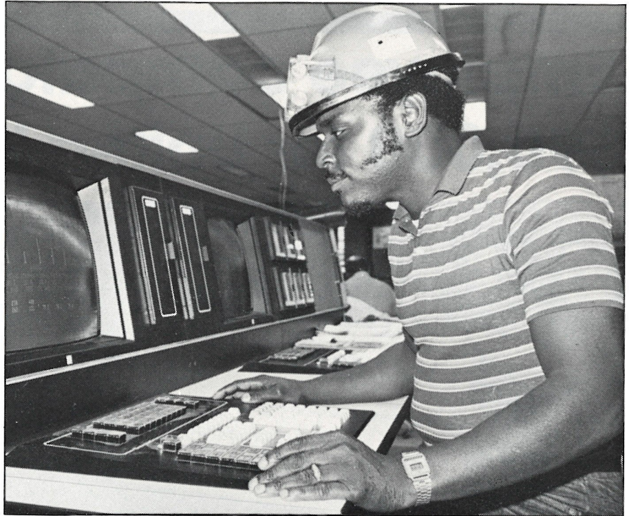
Raymond Tidwell, DU-2 operator, monitors thermocouple temperature readings at a Total Distributed Control (TDC) work station in the unit control room. Thermocouples were converted from control board instrumentation to TDC prior to the DU-2 shutdown. (See photo p. 6)
