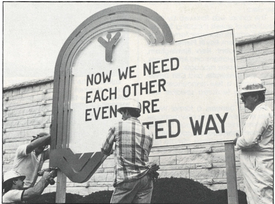
Up goes one of the four United Way signs built and painted by crafts employees to publicize the Complex fund drive. Installing the Main Gate sign are Bill Cerny, carpenter (lower left); Tim Richey, carpenter; Bob Johnson, laborer; and Roy Pickerill, truck driver. As of Oct. 12, employees had pledged approximately $72,000. Final campaign results will be published in the November Review.
