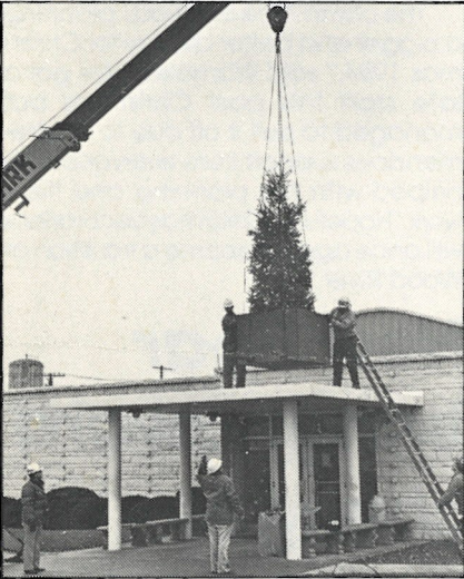
Up goes a live Christmas tree at the Cafeteria. Three others were placed at the Docks, Sulfur Plant and Field Office No. 1. The trees have since been planted at the Complex.
