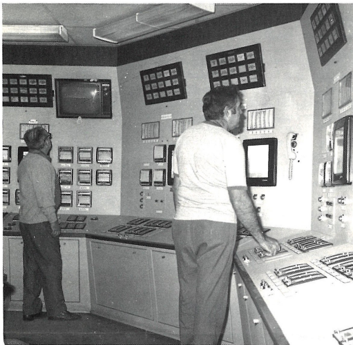
Virtually all of Utilities' activities can in some way be controlled or monitored from the Utilities Control Center. Here, Lennie Condellone, foreman, (left) makes sure boiler stacks aren't smoking by monitoring a closed circuit TV while operator-1 Jim Mussatto makes an adjustment to one of the boilers.
