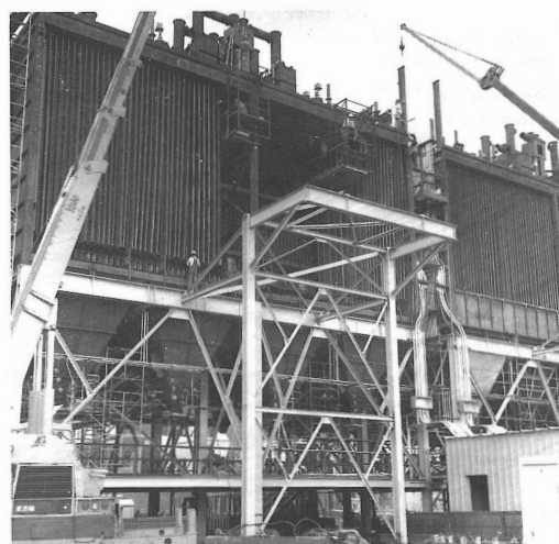
PRECIPITATOR CONSTRUCTION. Two electrostatic precipitators were built in 1975 to greatly reduce catalyst emissions from the cat crackers. Shown here are the many hanging plates that catch the catalyst by static electricity.
