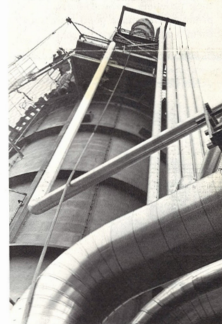
GLEAMING SILVER PIPES. H-7 furnace has been waiting since last spring to be tied into the CR-1 system. A good deal of planning and precise work went into this complex job.
