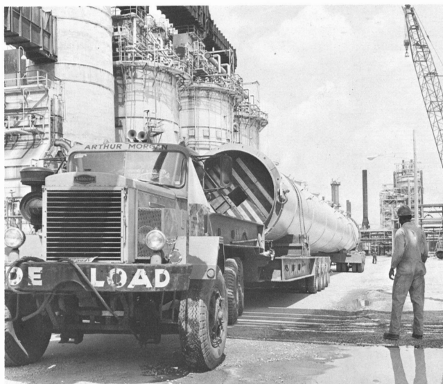
The massive lower section for the new cracked absorber is hauled from Alkylation to Gas by a special tractor trailer. The trailer alone has 56 tires. Assisting the driver maneuver his unwieldy load of 90 feet and 75 tons into place is Anton Williams, boilermaker helper.
