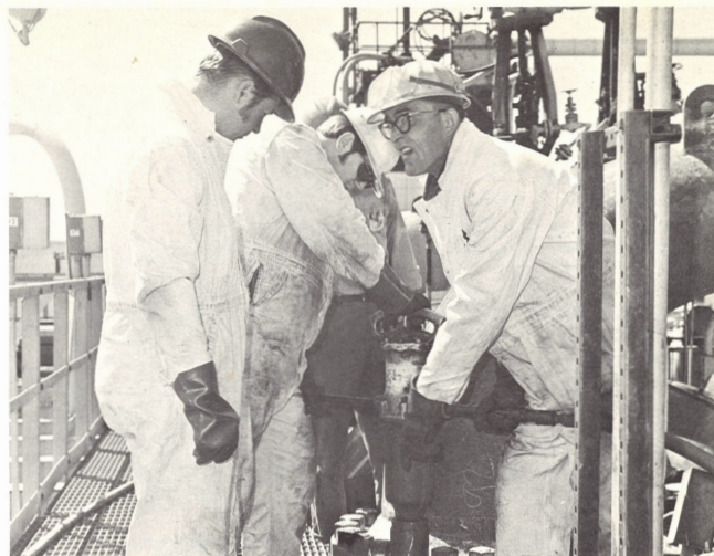
The final steps of a shutdown. In this case at the CR-3. While Don Perdun, boilermaker helper, looks on, Harry Kulp, boilermaker helper, and Dick Milcic, boilermaker 1st, use an impact wrench to head up a reactor.
