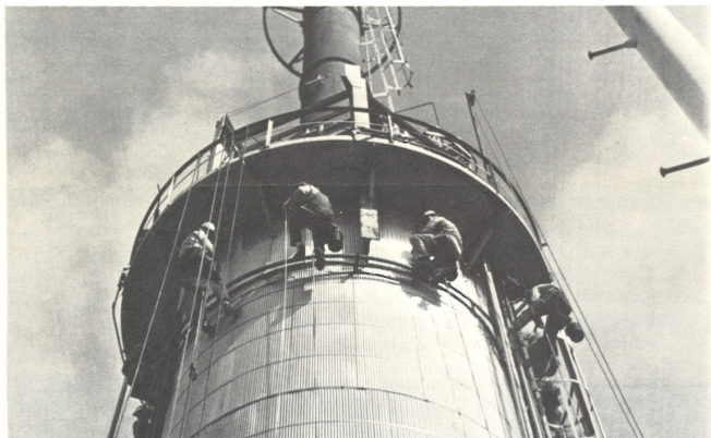
The Distillate Hydrotreater unit recently received a facelift in the form of a shutdown. These workers are putting the final touches on new insulation.
