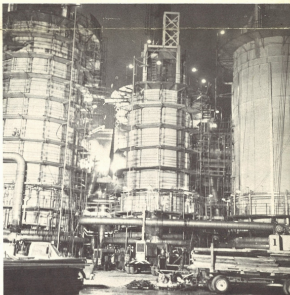
A nighttime view of the refinery in March, 1971. About 80 people a day, including men from virtually all crafts, worked night and day on two shifts through the weekends on a shutdown of catalytic reformer no. 3 in the Aromatics department.
