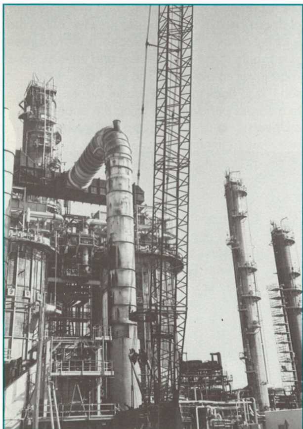
Positioning a new convection section atop DU2 required the help of large cranes.
