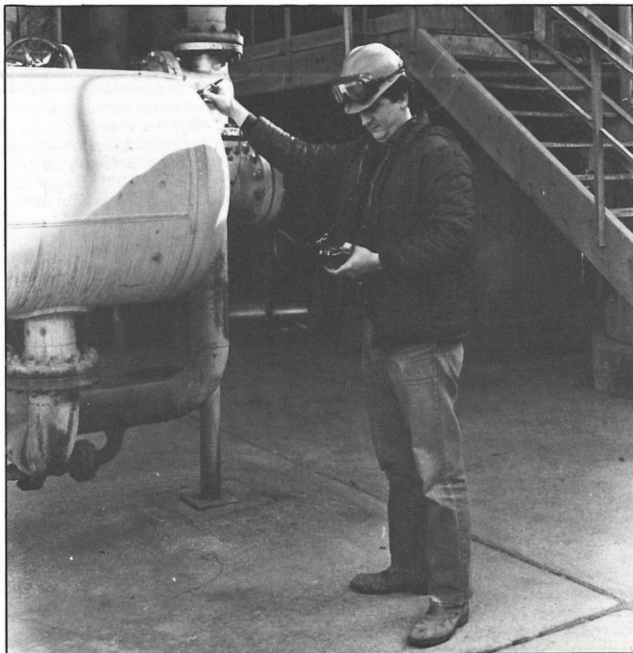
Randy Fickert, pressure vessel inspector, tests an exchanger shell in CCU-1 for corrosion. Inspectors are responsible for monitoring pressure vessel equipment for defections specifically, corrosion.
