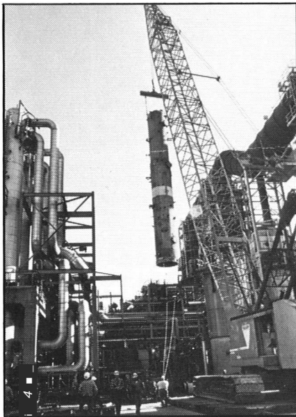
Up, up and away!!! CR-1's 60 foot, 35,000 pound caustic water wash column is lifted from its foundation.
