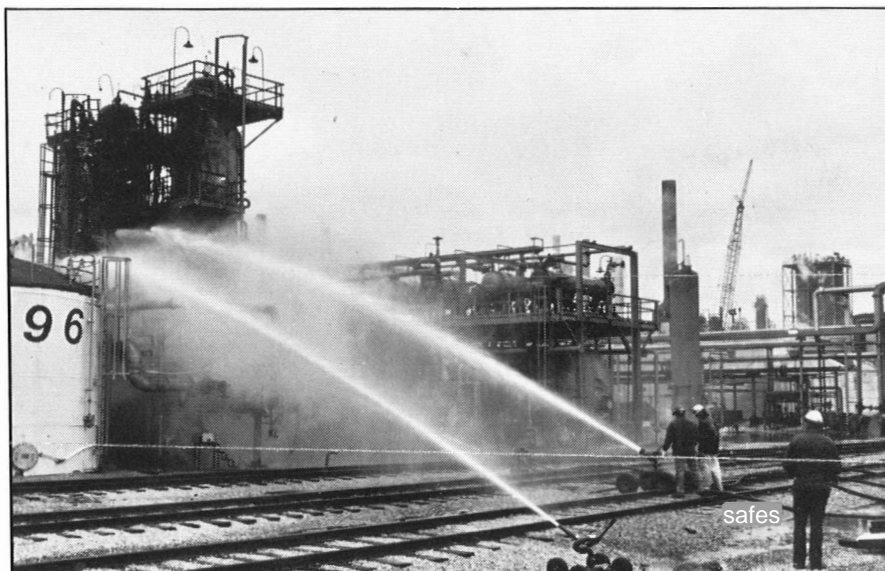
Water streams are directed on the D&D unit after explosions and fire occurred Jan. 23. Shell's Fire Crew had the blaze under control within two hours which prevented further injuries or damage to nearby equipment.
