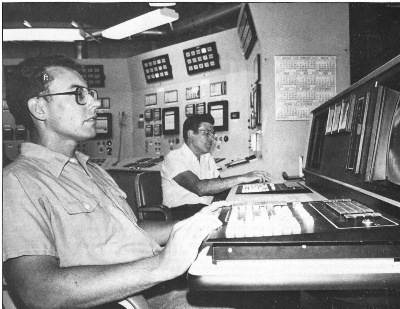
Working with a new Total Distributed Control (TDC) system at the Utilities Control Center are Ron Smith, energy systems operator (left), and Earl Nallor, boiler operator. TDC is replacing the boiler control boards shown behind the operators.
