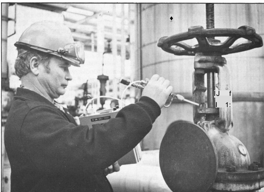
Paul Sibley, operator at Aromatics East, uses a detection instrument to test a CR-3 valve for vapor leakage. Approximately 31,000 Complex valves, pumps, compressors and process drains are regularly monitored for liquid and vapor emissions; those that leak are repaired.
