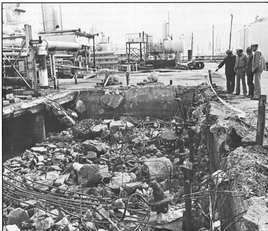
After about 25 years of service, the Sulfur Plant D pit is being completely renovated. D pit is used to contain the liquid sulfur recovered from petroleum by the Claus units. The sulfur is sold to industrial customers. (Photo by Randy Millikin)
