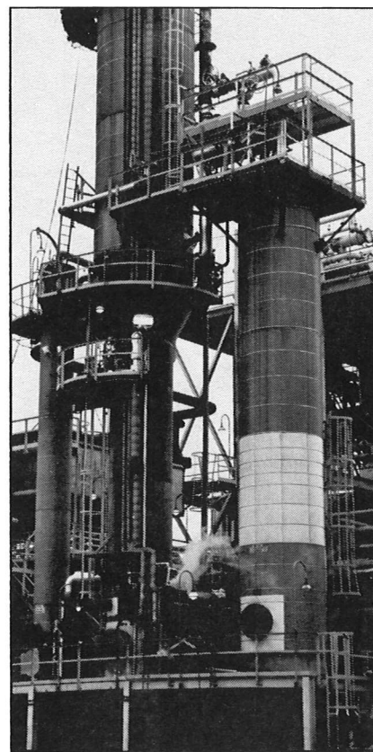
The Visbreaker converts residue into lighter fractions. It was started up in November as part of WRMC's residual yield reduction program.
