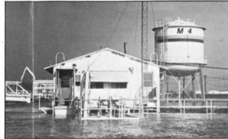
At its highest flood level the river was six inches from the dockhouse floor. The dockhouse sits on a steel structure 15 feet above ground.
