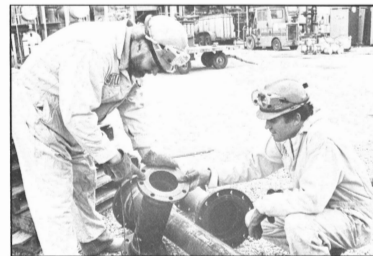
Below: Inspectors Bill Jacobs and Ron Baggett examine the gasket surfaces of new pipes for Cat Cracker-2.
