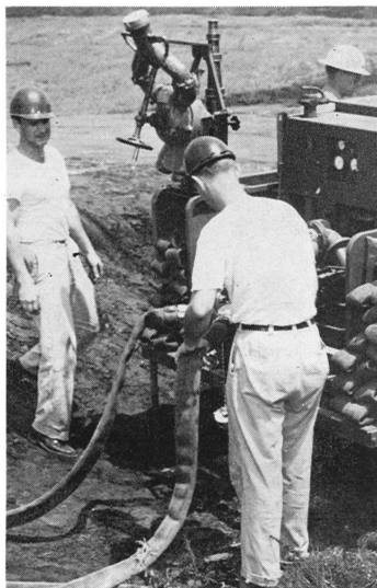
A new addition to the refinery's fire-fighting equipment is the Hale booster pump, which is able to force water over the highest tower in the plant. This pump can boost regular refinery water pressure to reach high elevation. It is used in conjunction with a portable turret nozzle.
