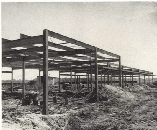
Looking east, steel structure for the new Maintenance Shops building appears to be almost complete. The new building will resemble Stores in architecture, will be only 30 feet high. The Instrument Shop and offices will make up the southwest corner of the building in the foreground.
