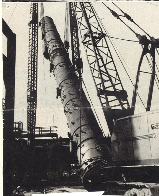
Over-all size of the column can be appreciated when compared to man standing above. He is checking all lines attached to the column. Five-sheave blocks hold cables in place.
