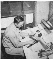
C. A. MARTIN, Machine Shop draftsman, is measuring a shaft sleeve preparatory to drawing it. Martin drafts models for the shop files.
