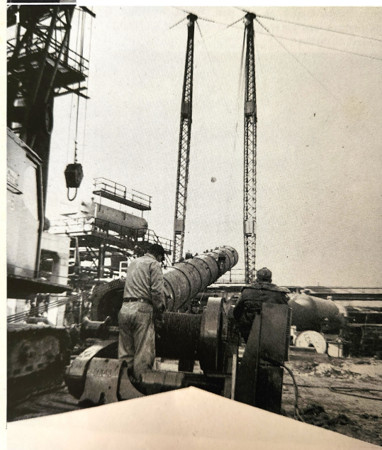
This operation had to be performed before the column could swing between the gin poles. These men are securing cables to the base of the column prior to final alignment preparatory to completion of erection.
