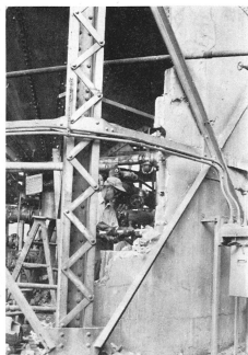
A brick skirt around the agitator had to be torn down. The skirt was 15 feet high, and had stood since the day the agitator was built. Most of this work had to be done with a sledge hammer.
