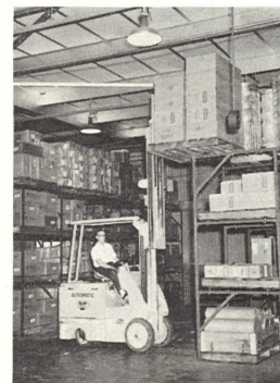
Fork lift trucks are used to stack and remove material from the storage racks. All bulky materials are palletized to make this type of operation possible. Operating this lift is Counterman R. M. Neely.
