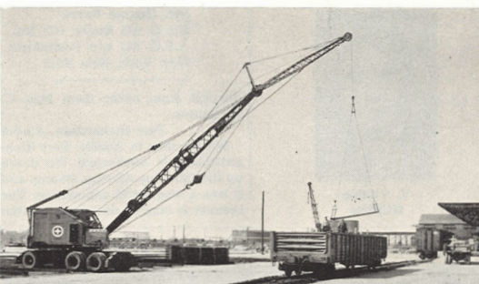
A crane removes tubing from a railroad gondola car and stacks it on the timbers placed in the yard for this purpose.
