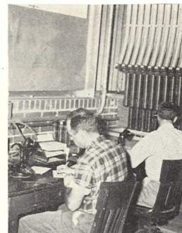
Calls for material are received at this station and orders made up and dispatched through the pneumatic tube system, part of which is shown at the right. Countermen L. Vander and R. M. Hester are at the desk.
