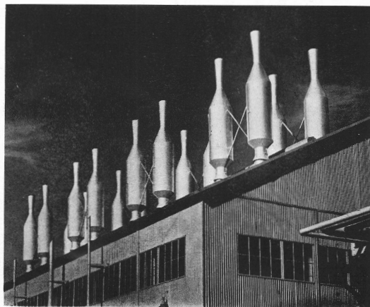
These silvery objects are neither giant bottles nor oversize bowling pins, but compressor exhaust mufflers on the roof of a Shell Oil Company gasoline plant at Wasson, Texas. The plant processes natural gas produced along with crude oil. Valuable liquid gasoline components are recovered, and the dry gas is used for cooking and heating.
