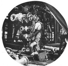
A pipefitter dismantles the valve manifold of Agitator No. 2 preparatory to hauling the treat-upto the salvage yard. This was a large operation. All pipes and connective lines had to be removed before the old agitator could be hauled away.
