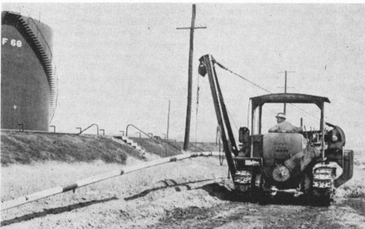
The side boom crane assists with the laying of pipe in North Property. The operator is A. Sharleville.
