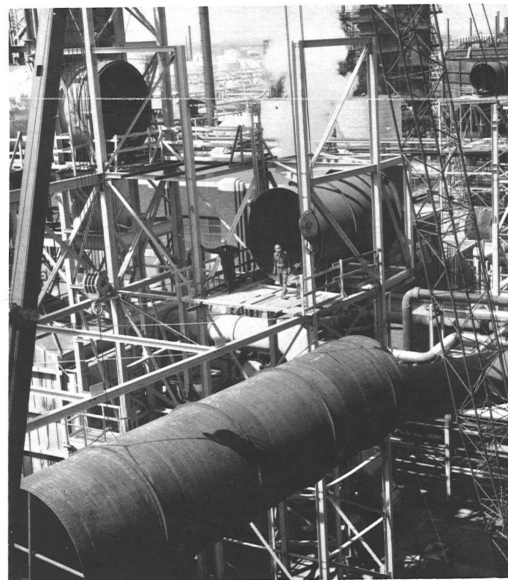
TIGHT FIT. During construction Shell boilermakers and cranes combine to set a 40-foot piece of precipitator duct 65 feet above the ground. They had all of one extra inch of space in which to maneuver it into place! Whitey DeLassus directed the effort.
