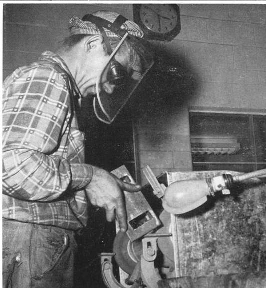
MOST EMPLOYEES , like Valve Repairman A. E. Culp, are conscientious about safety on their jobs here at the refinery. Culp uses a safety shield while using the emery wheel at Shops One. Employees should be just as safety-conscious at home, where accidents can happen without warning.
