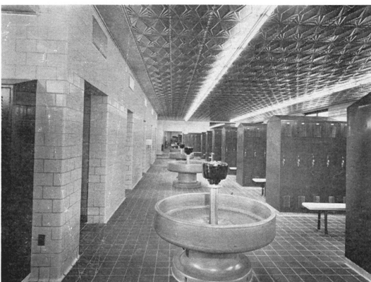
AN AISLE VIEW of the new addition shows four Bradley wash stands, each of which can serve eight employees at one time. New metal lockers can be seen in banks at right. Metal ceiling was required to resist high humidity conditions.
