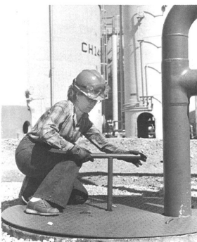
A QUICK TWIST of the valve by Elouise Whitlock, operator helper, Aromatics-East, starts the heavy spray at the DHT truck rack several yards away.
