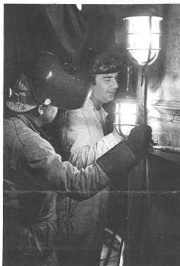
TEST FOR PERFECTION. Frank Pinkas, Engineering Services inspector, gives the OK to a weld made by boilermaker Don Carpenter.
