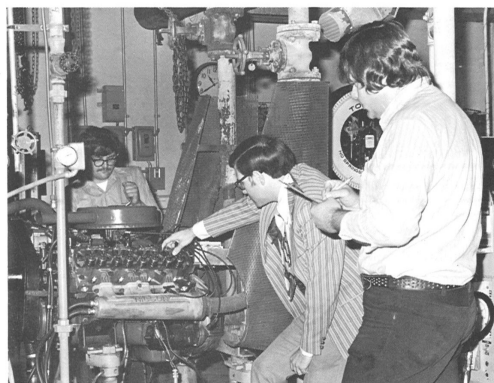
TEST RUN. As research mechanic Fred Windisch removes the second valve cover, research engineer Don Evans makes a preliminary check for deposits of wear, and Floyd Albert, senior lab technician, makes note of their impressions. All three have been closely associated with the testing of lubricants.
