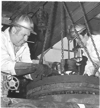
'BATTEN THE HATCHES'. Boilermaker Joe Strayhorn and boiler helper Gary Arth prepare a CO-5 exchanger for a tubular test.
