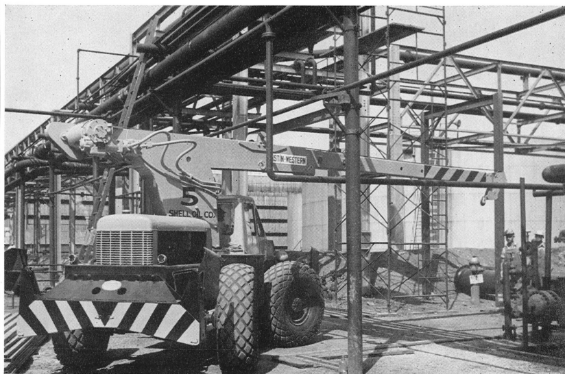
Wood River Refinery's new hydraulic crane, capable of maneuvering in small areas, here lifts cooling water lines into place. The crane is particularly efficient in low-ceiling areas, as it has a clearance of 10 feet, 6 inches. The unit has a telescopic boom, and is capable of lifting 5 tons. It has power-steering and can move at a 30 degree angle sideways.
