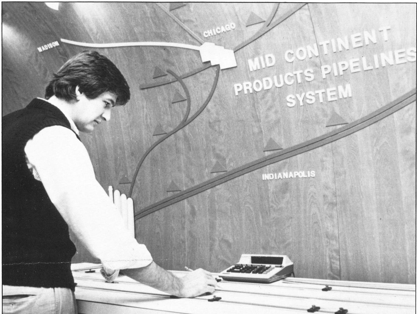
Mark Bowen uses a "paper pipeline" to track movement of products through the five outgoing pipelines from Wood River. Bowen, a Shell Pipe Line controller, can determine nearly exact product arrival times at the 12 Distribution Plants located along the pipeline system.
