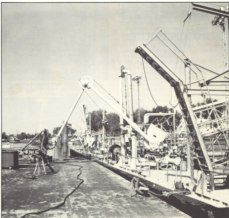
The Shell docks are a place where an ounce of spill prevention is the cure.
