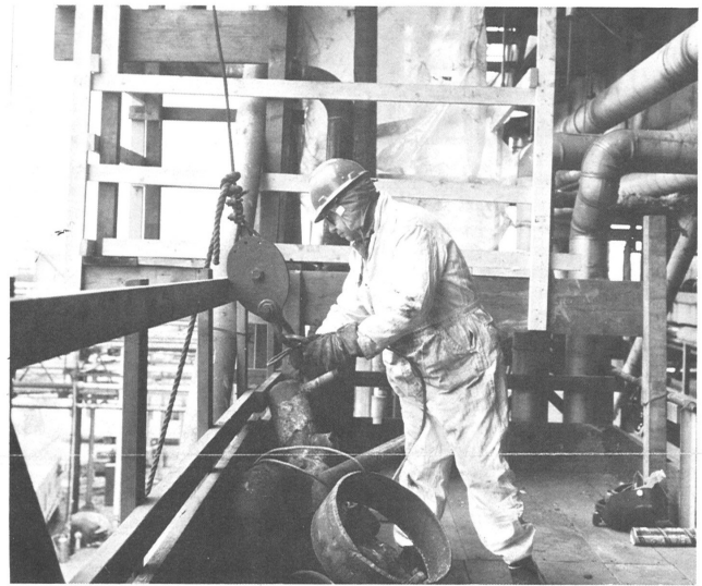
Gene Benner, Pipefitter 1st, at work during the Cat Cracker shutdown.
