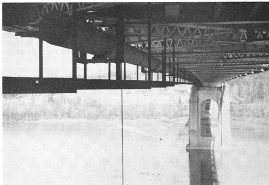
ACROSS THE WIDE MISSOURI stretches this section of Shell Pipe Line Corporation's Ozark System, recently put back into operation following re-routing. The 22-inch line was suspended beneath the deck of the Daniel Boone Bridge across the Missouri on Highway 40 west of St. Louis. This photo was taken while contractors still were working on the pipeline and approaches to the bridge.
