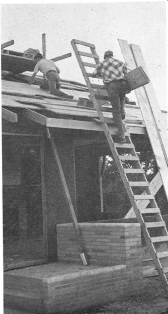
ABOVE, This picture, taken two weeks after the fire, shows the progress being made on the house. All the siding has been nailed on, the floor rebuilt and the roof is nearing completion.
