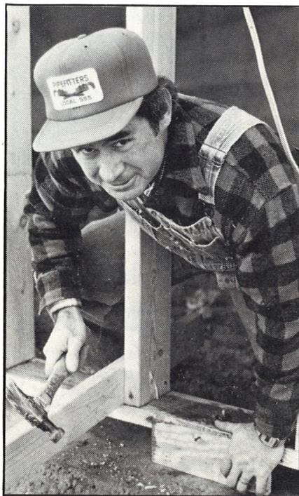
One of the most reliable Shell volunteers is Larry Fencel, a pipefitter. He said he strongly believes in the value of the Teen Challenge program.
