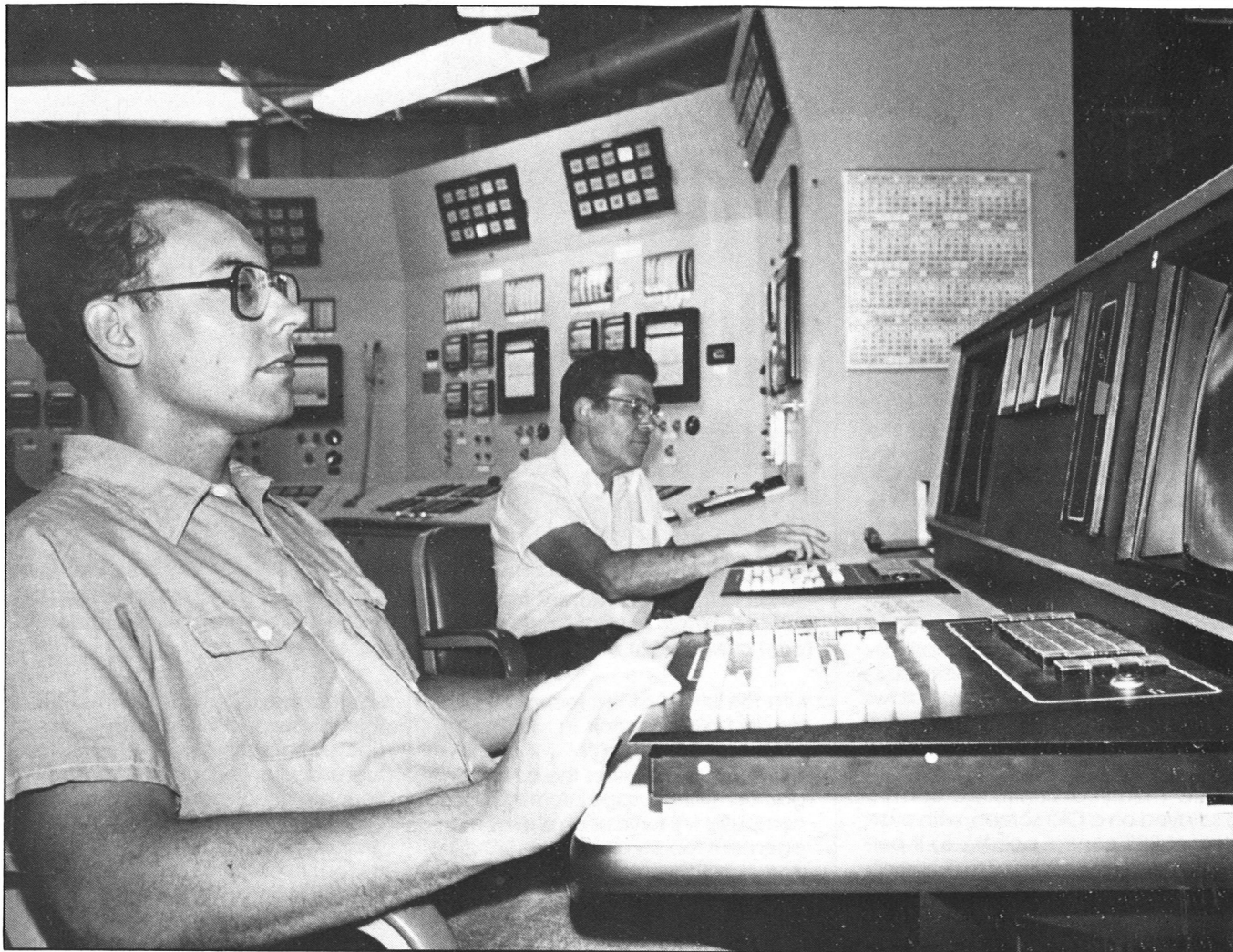
Working with a new Total Distributed Control (TDC) system at the Utilities Control Center are Ron Smith, energy systems operator (left), and Earl Nailor, boiler operator. TDC is replacing the boiler control boards shown behind the operators.
