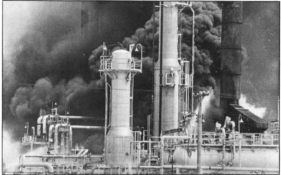
Smoke billows from the Kerosene Hydrotreater Unit during a fire on June 26. The Fire Crew promptly responded to the emergency and extinguished the fire in less than an hour. The fire broke out when a 12-inch process line failed and the leaking product ignited. (Photo by John Badman, Alton Telegraph)
