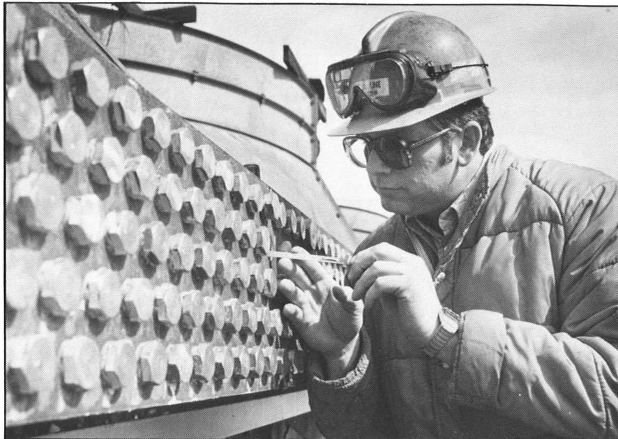
Denny Line, senior inspector, checks the condition and consistency of threading on low-temperature shift effluent air coolers at the Steam Methane Reformer. Line is assigned to the Engineering Support group of Major Projects.
