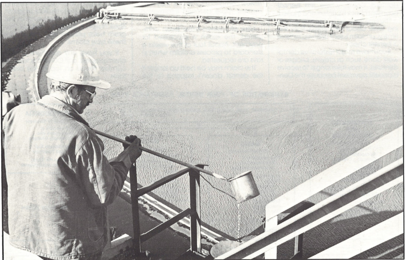
Leroy Edwards , Utilities operator, takes a waste water sample from Dissolved Air Flotation Unit No. 2 at the Waste Water Treatment Plant. Samples are tested to determine the levels of phenol, ammonia and sulfide, and the pH.
