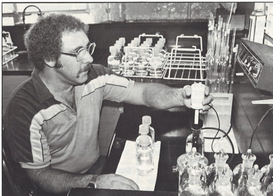
The Quality Assurance/Environmental Conservation Lab tests about 200 process waste water samples each week. Results of these analyses are sent to the Illinois Environmental Protection Agency. Above, Wayne Michalik, special tester, performs a bio-chemical oxygen demand analysis to find the level of organic contaminants in Complex waste water.
