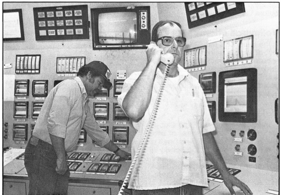
Tom Rock and David Webb, operators at the Utilities Control Center, are shown next to the boiler control panels that will be replaced next year with computer terminals. The new computerized system will run the Complex boilers, generators and steam letdown system. Operators will make adjustments by keyboard instructions and "touch" screens.
