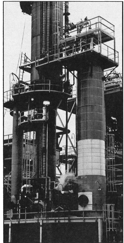
The Visbreaker converts residue into lighter fractions. It was started up in November as part of WRMC's residual yield reduction program.
