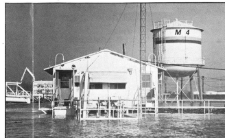
At its highest flood level the river was six inches from the dockhouse floor. The dockhouse sets on a steel structure 15 feet above ground.
