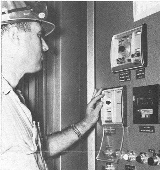
ADJUSTING CONTROLS on the console of the new asphalt blender in the Lubricating Oils Department is Operator 1st Adolph W. Borgini. The new equipment blends asphalt compositions as required, mixing materials from two tanks in the proper ratio while loading in railroad tank cars or trucks.
